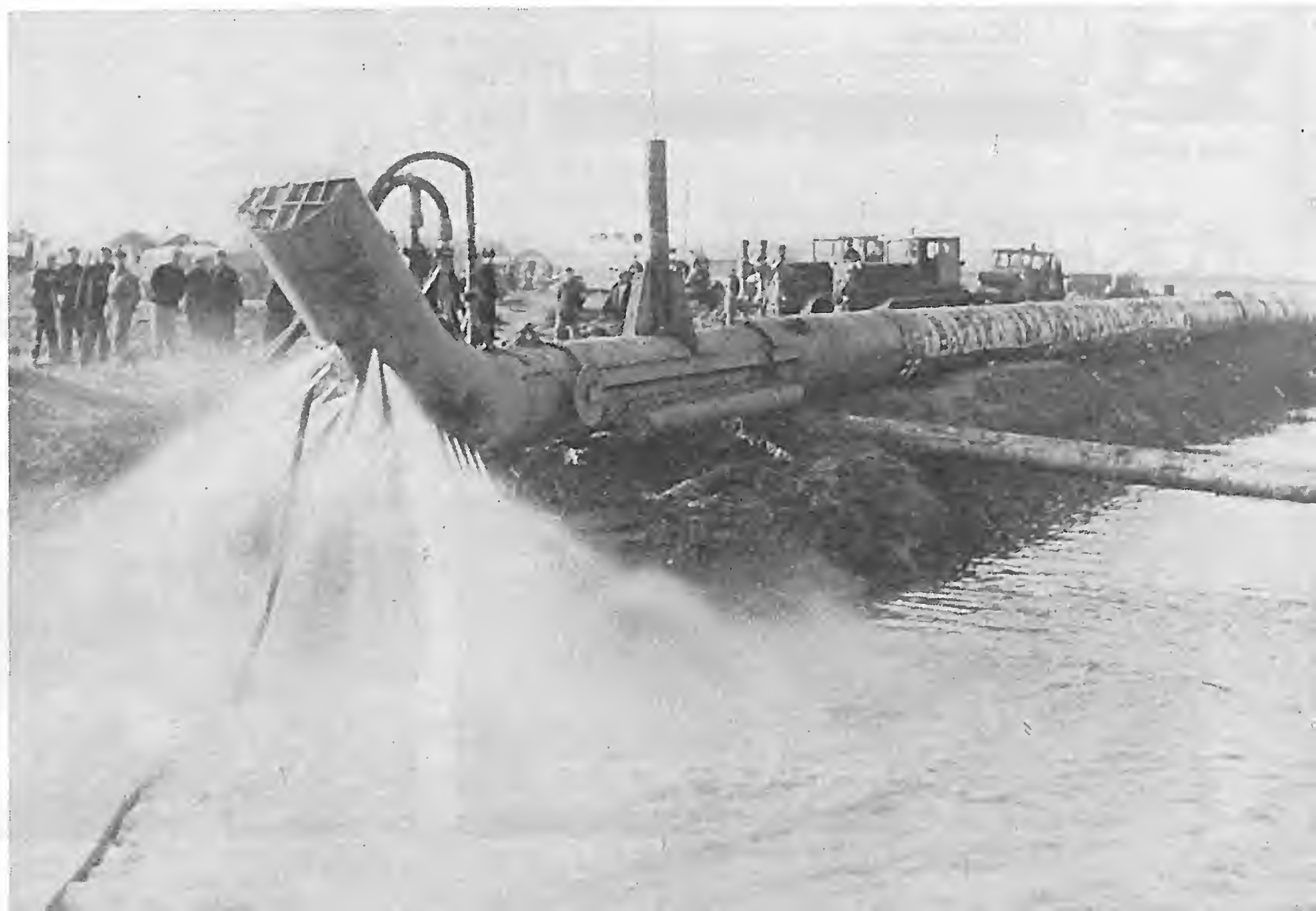
The pipeline being laid on the bed of the Nunkiang River.
